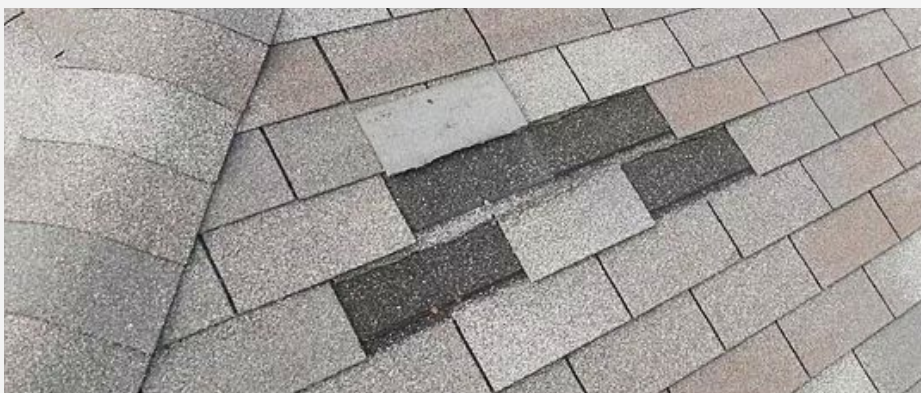
MISSING SHINGLES
